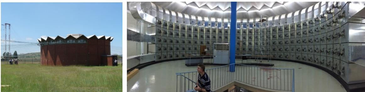
The outgoing feeders from the transmitters converge upon the antenna switch via four massive subterranean tunnels. The switch connects any transmitter to any antenna via open wire feeders (none of your 50 ohm nonsense! photo by Riaan ZR6VAN). The intrepid Kevin checks out the basement for any unattended spare parts.
