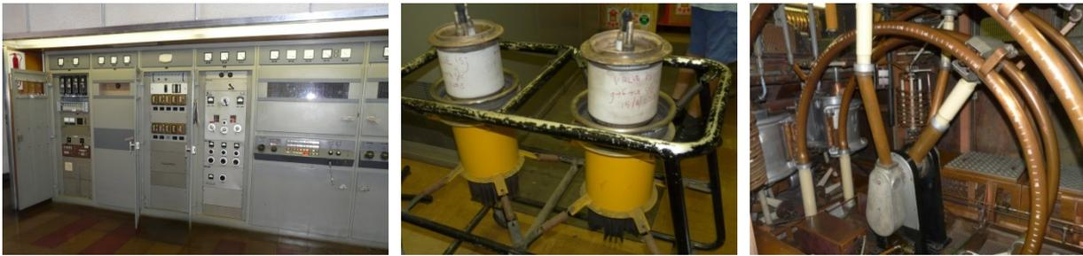
L to R: The Brown Boveri 200kW transmitter, its water cooled valves, and a rotary inductor to die for!
