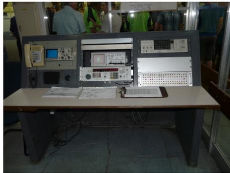
L to R: The ADSL links where the audio arrives, Kevin ZS6KAT adjacent to the audio patch board standing Guard over the Revox Tape recorder used for programme intermissions covered by Rad ZS6RAD, and the central monitoring desk for all outgoing transmissions.
